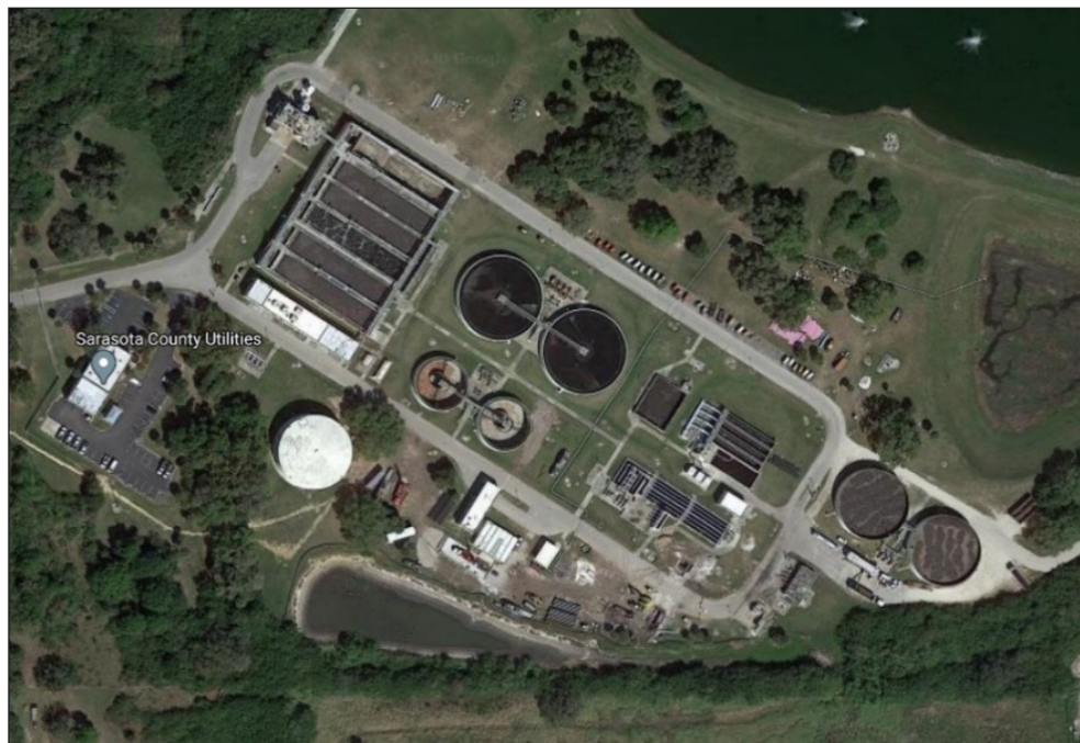
Figure 1. An aerial view of the facility.
